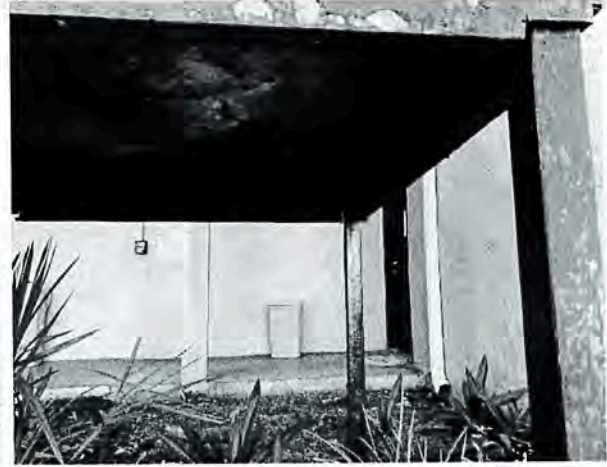
Photograph 14: Common areas staircase landing and columns
