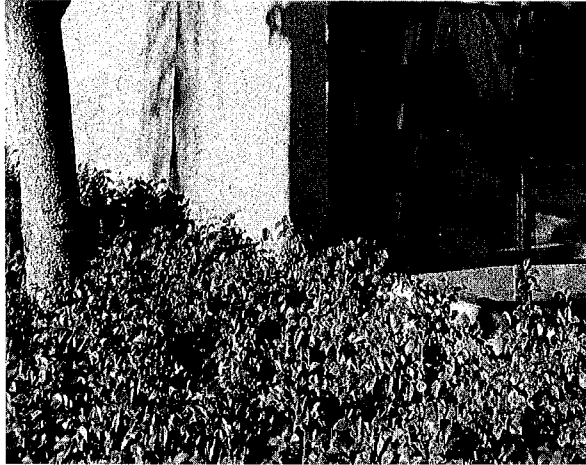
Photograph 13: Tree root growing against the foundation
