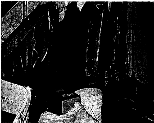
Photograph 9: Unit 204. Household item within the attic space
