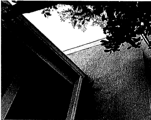
Photograph 11: Opening in the exterior wall
