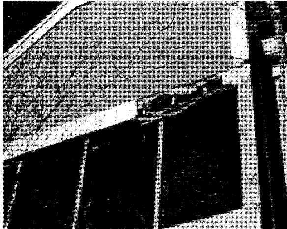
Photograph 15: Opening in the exterior wall
