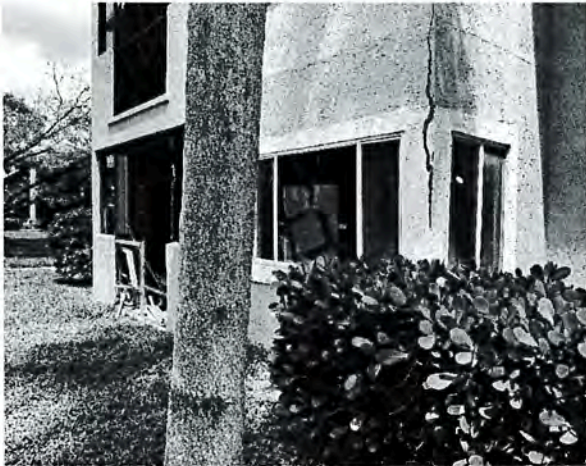
Photograph 1: Building elevation Blue Tarp required
